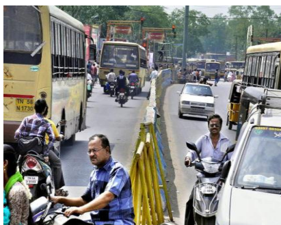
Figure 4: Issues in Traffic, Parking & Pedestrian crossing in Madurai CBD
